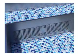
Unique to Bradford Spas is the stainless steel collection port. This reduces the number of visible fittings and drain covers in the spa foot well.
